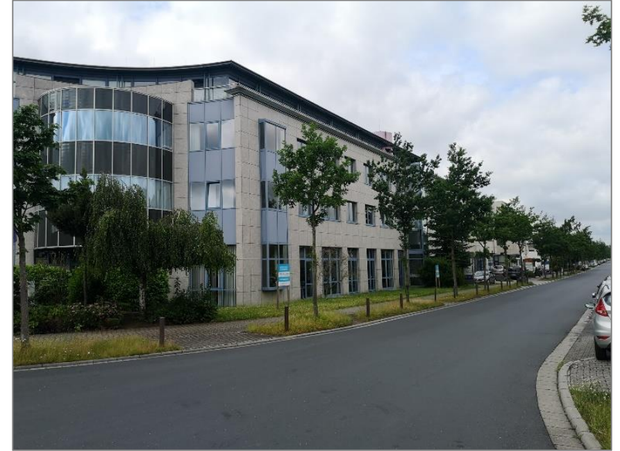
R&D Office, Germany
