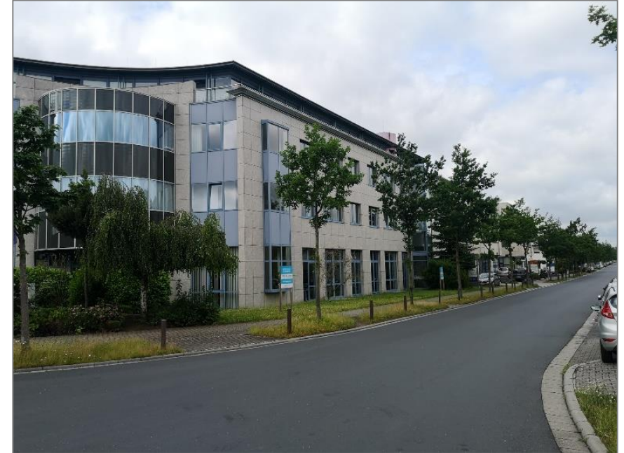
R&D Office, Germany
